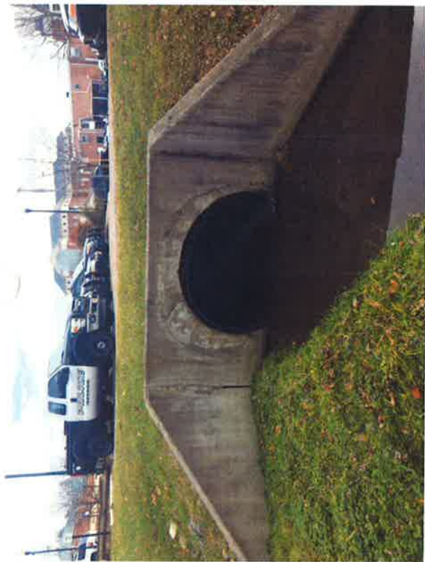
Police Station culvert outlet
