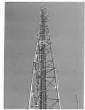
A Greenfield-type tower used in base stations for mobile telephony
