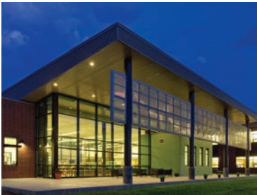
Blacksburg High School (PPEA)
