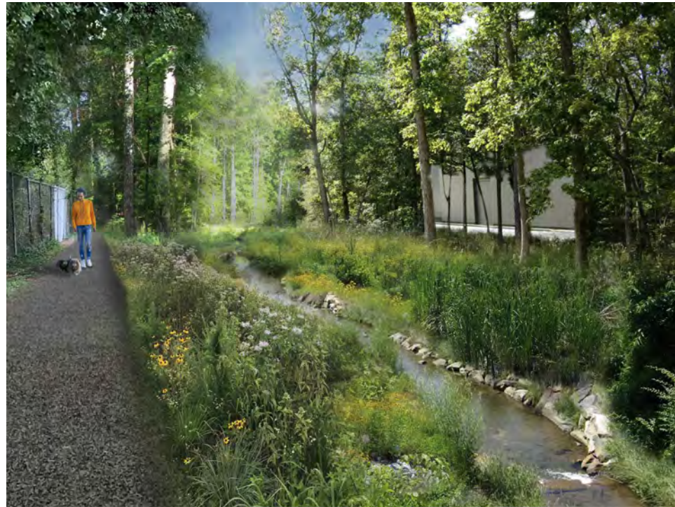
RENDERING OF RESTORED CHANNEL WITH MODIFIED CROSS VANE AND DENSE RIPARIAN PLANTING.
