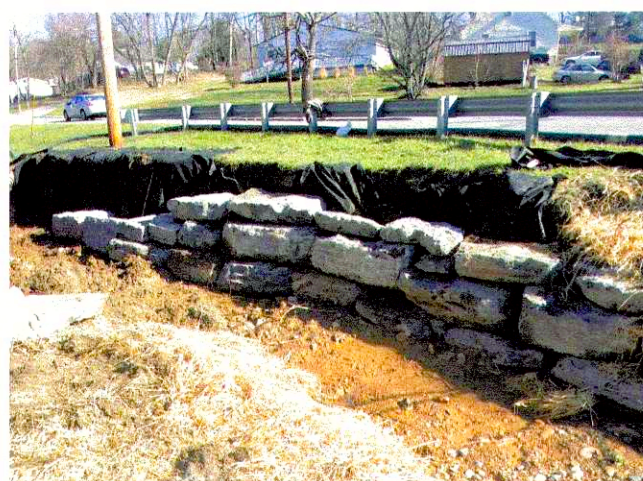
This photo shows the construction of the stone wall to repair the eroding stream bank along Depot Street.
