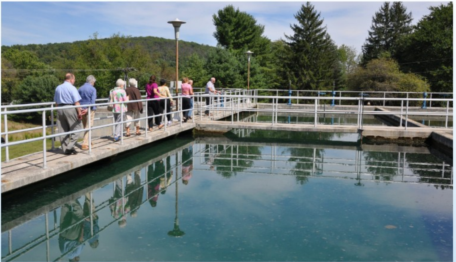
Above: Residents tour the sedimentation basins at the NRV Regional Water Authority's treatment plant.
