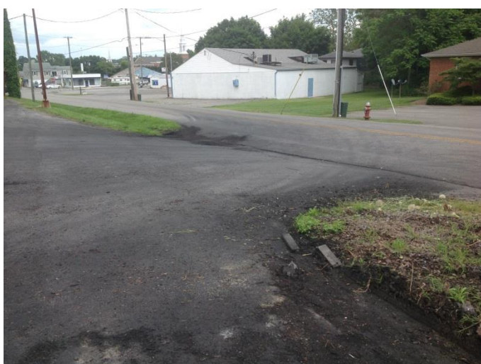
Photo 3. June 2, 2016 Site Visit. Verified material cleanup.
