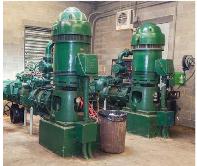
Pictured are two of the plant's water pumps. The pumps draw water from the New River to the treatment plant.
