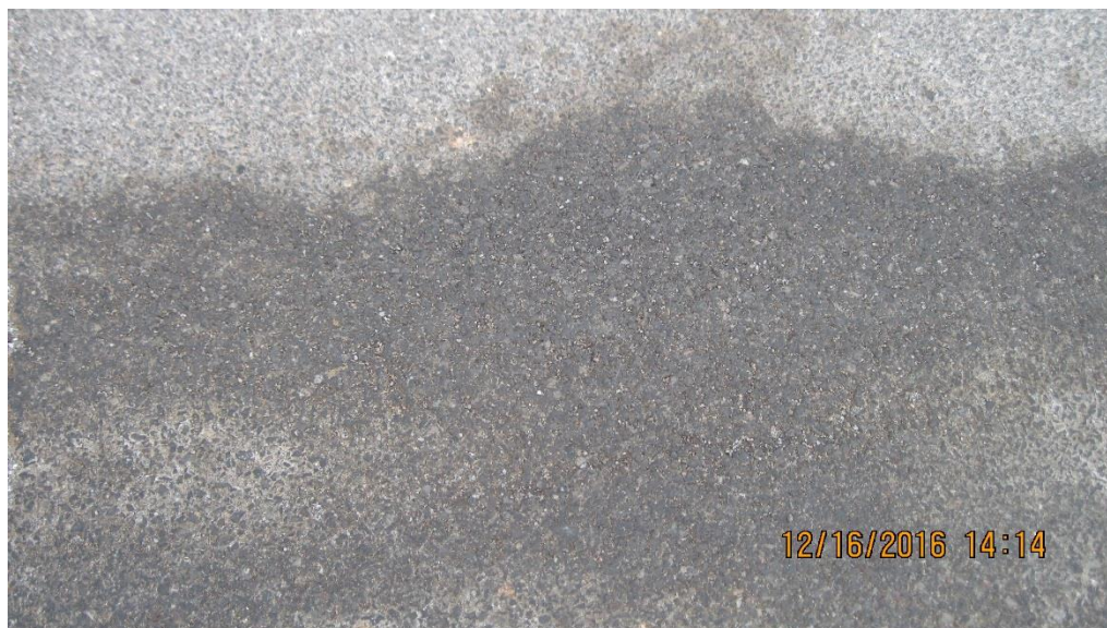
Photo 2. December 16, 2016. Close up of hydraulic line spill after sorbent application.
