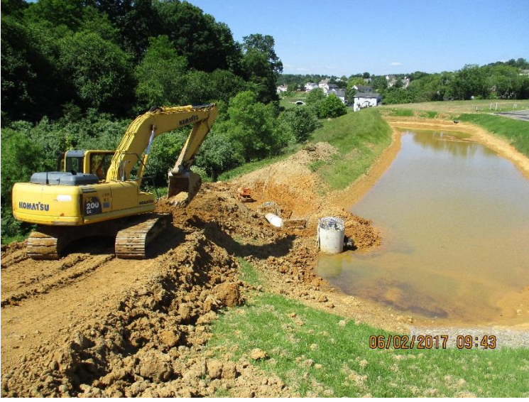
Photo 4. 6/2/17. Concrete cradle installation
