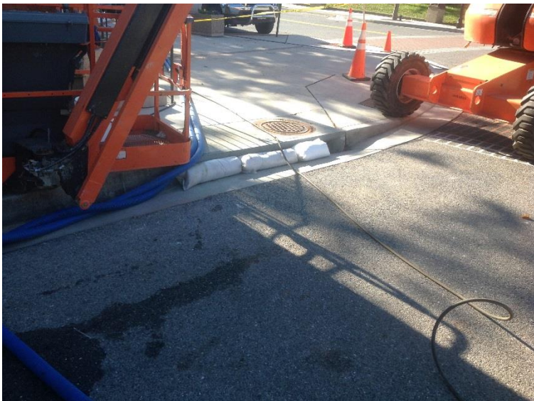
Photo 1. October 24, 2016. Storm drain inlets are protected from possible spills.
