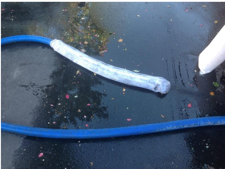
Photo 2. October 24, 2016. Suction line with filter sock to collect power washing runoff.
