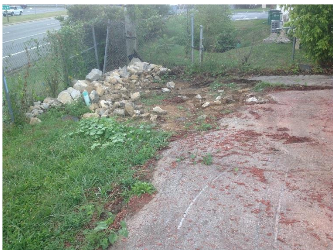
Photo 2. September 19, 2016. The potential for material discharge was observed and discussed with the owner.
