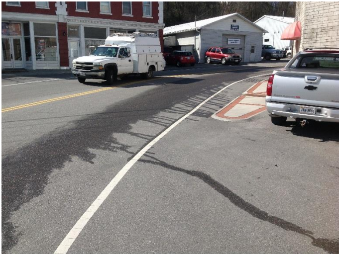
Photo 1. 3/20/17. Excavation to inspect manhole outlet pipe.
