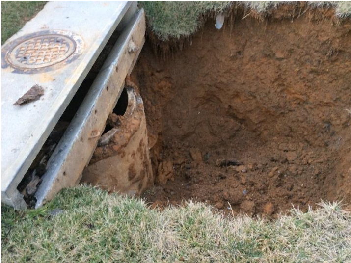
Photo 1. 1/24/17. Excavation to inspect manhole outlet pipe.
