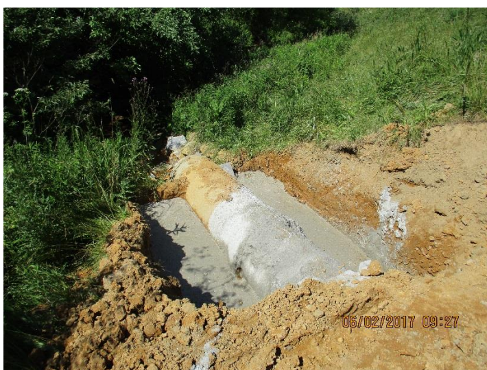
Photo 3. 6/2/17. Concrete cradle installation
