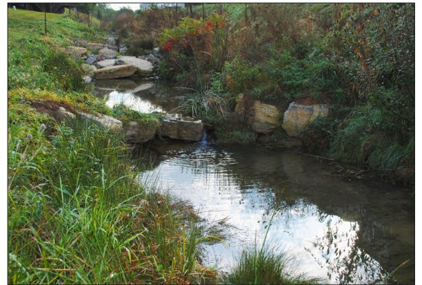
A portion of the restored stream near Blue Leaf Drive.
